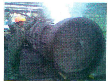
Picture 9 Cleaning of the heat-exchanger shell-side by HP water supply
